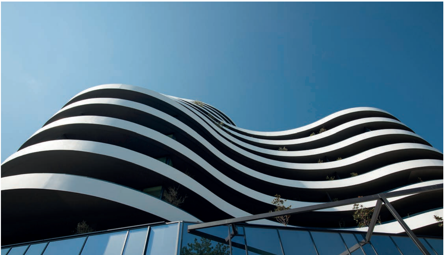
RESIDENTIAL BUDVA / Budva - Montenegro Architecture: Branislav Mitrovic and Jelena Kuzmanovic - Photography: Slaven Vilus
